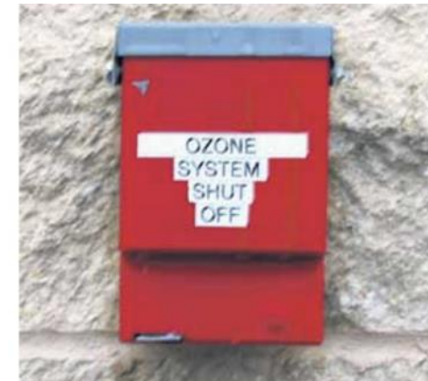
Ozone generator emergency shut-off should be located OUTSIDE the generator room!
